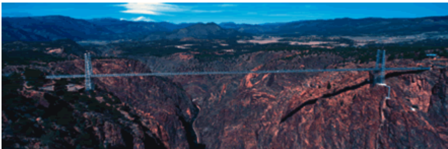
The Royal Gorge Bridge (built 1929) near Cañon City, Colorado, is the world's highest suspension bridge, with length 384 m (1260 ft) and width 5 m (18 ft).
